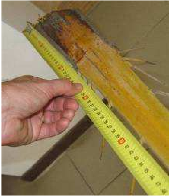
Installation of the tape measure
